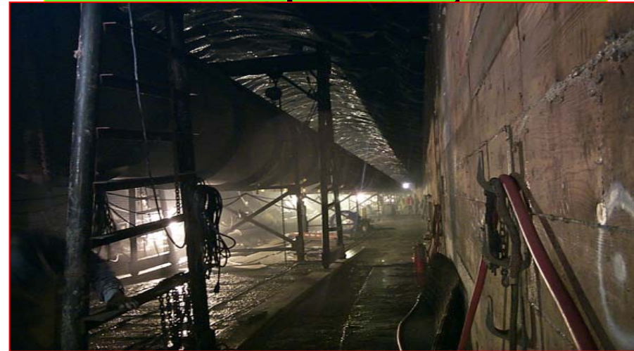
Decay pipe is finished and
