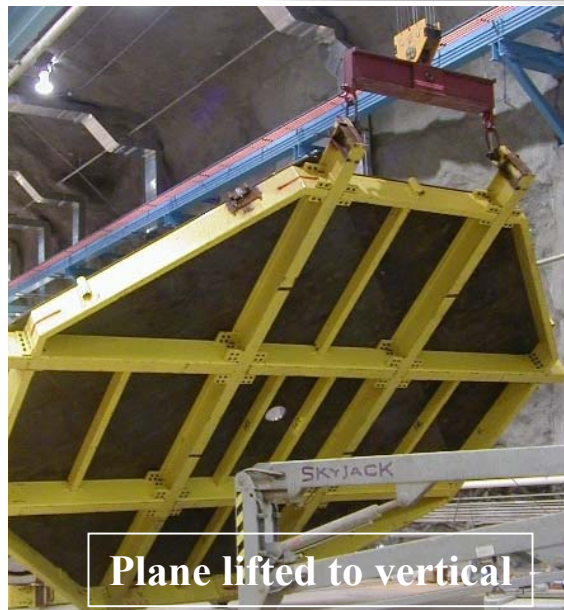
Crane carries plane down the hall for installation
